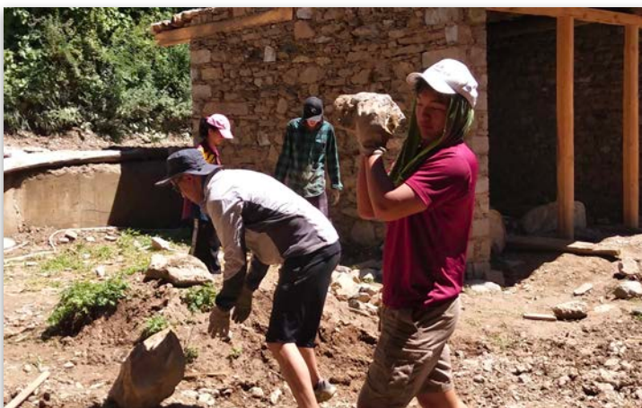
Moving rock and earth for construction
